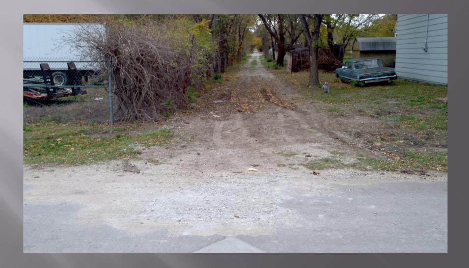
Dug up abandoned service in the alley □ CGI in the banks of the ditch line ■ 90% gas in all directions Proceeded east along sewer ditch Continued to CGI-high readings Dug 125' Uncovered blowing gas □ 2″ main cracked
