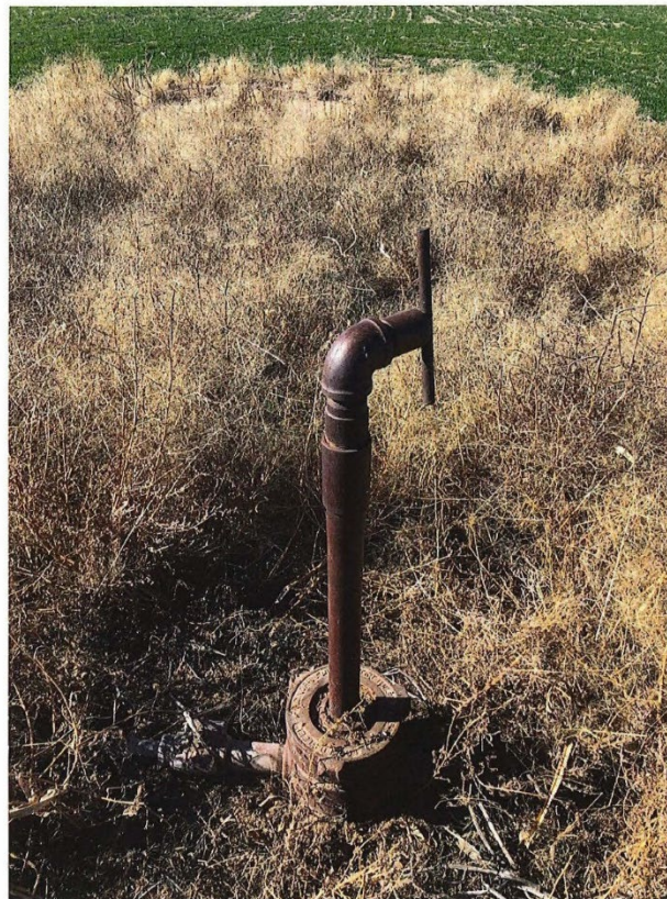
11/19/2020 Lemert Twin #1 SW 4-T35S-R34W Seward County, Kansas
