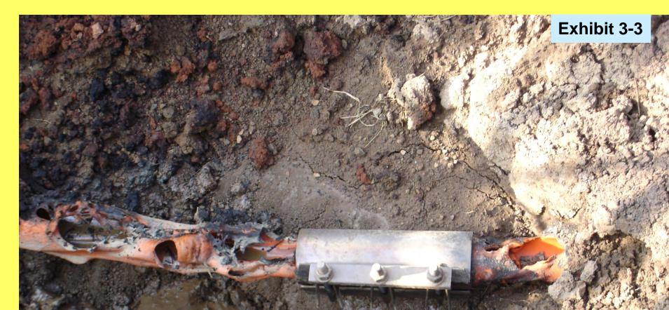
Damaged pipeline showing Clamp that was to be installed over leak
